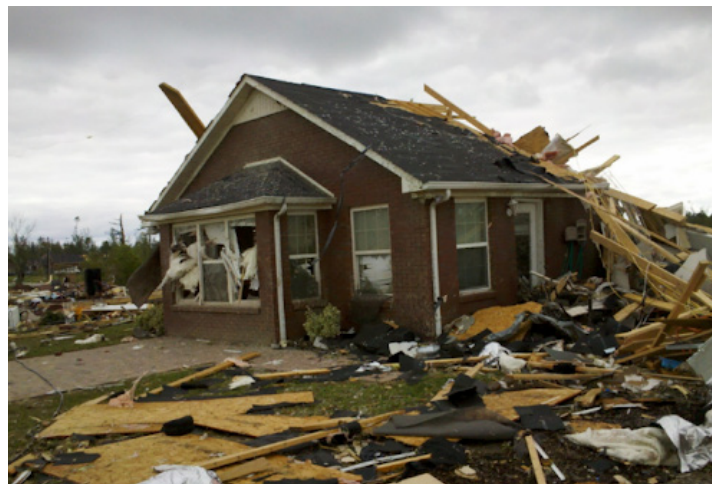
What was left of the Harrisons' home
