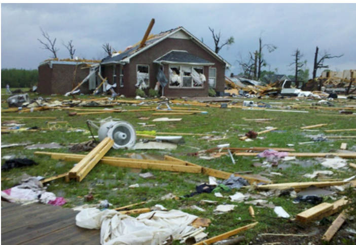
Devastation shown from the back of the home
