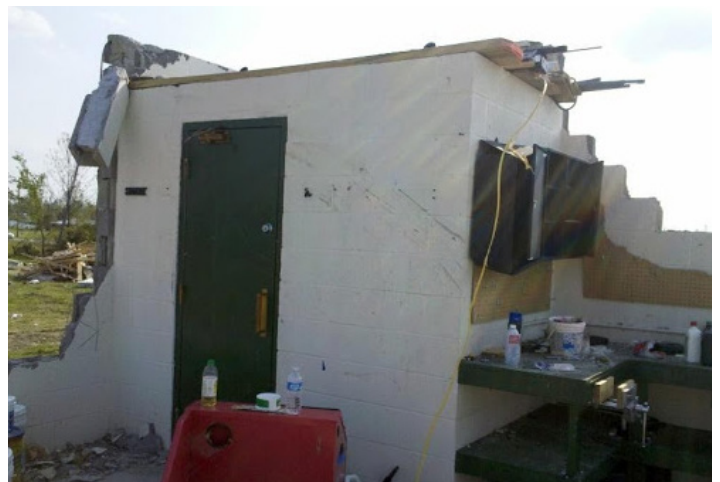
The tornado safe room: all that was left standing of the Harrisons' garage
