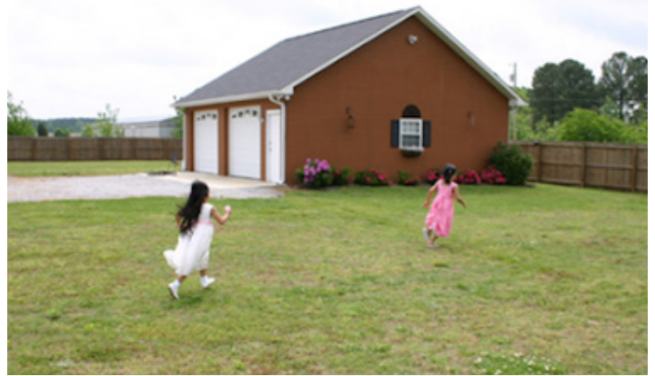
Garage that contained the tornado safe room
